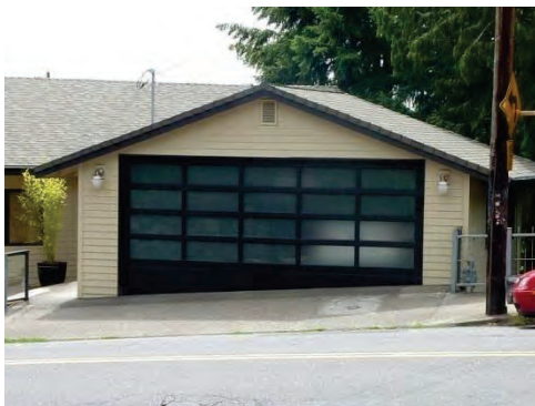
An Inappropriate Mostly Glass Garage Door
