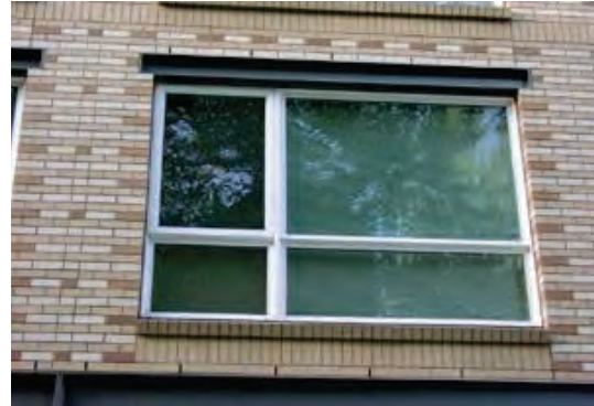
Example of Non-Complying Window, With a Vertically Asymmetric Division
