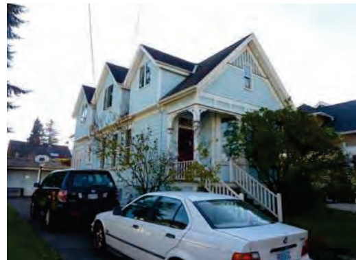
Examples of Excessive and Out-of-Scale Dormers
