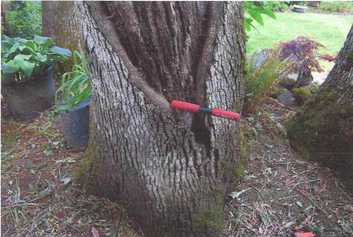
View of west tree on east side with probe 4' into cavity.
