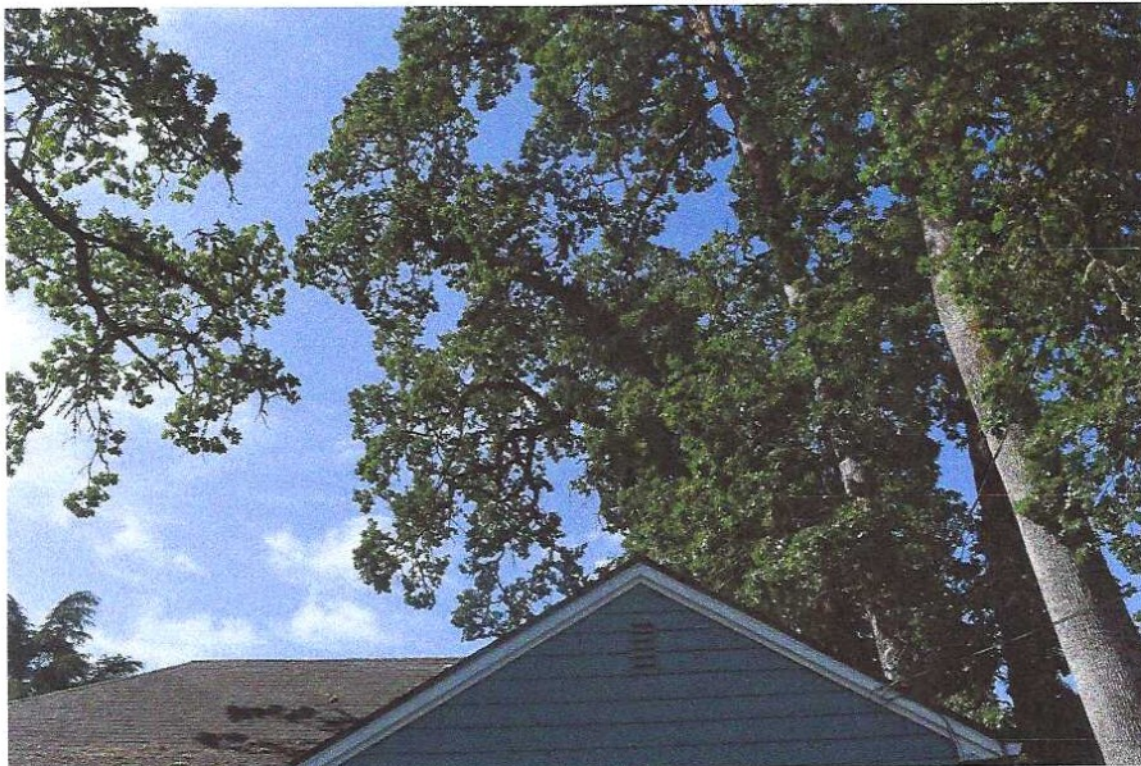
View of the tree behind house with hard lean over house.
