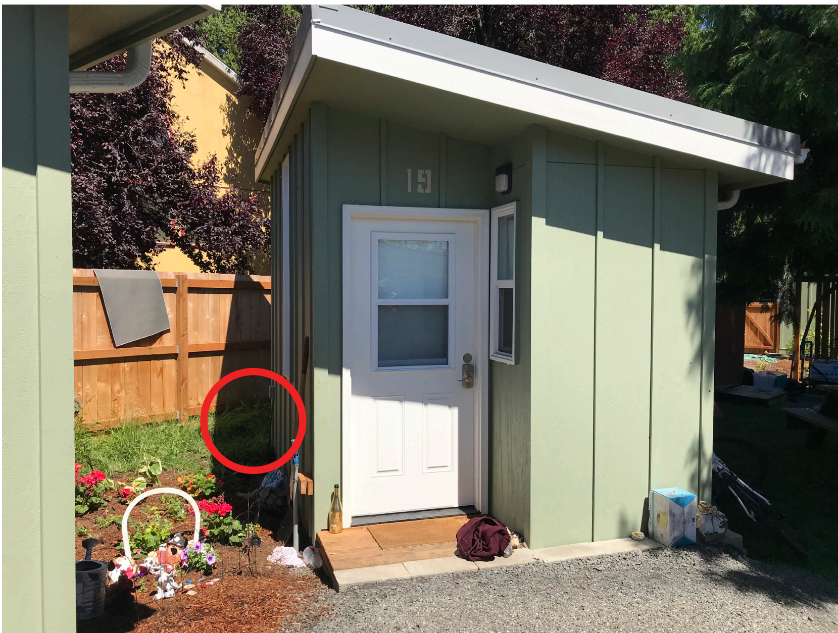
ELECTRICITY HOOK-UPS AT THE ST. JOHNS VILLAGE MINIMIZE VISIBLE WIRES
