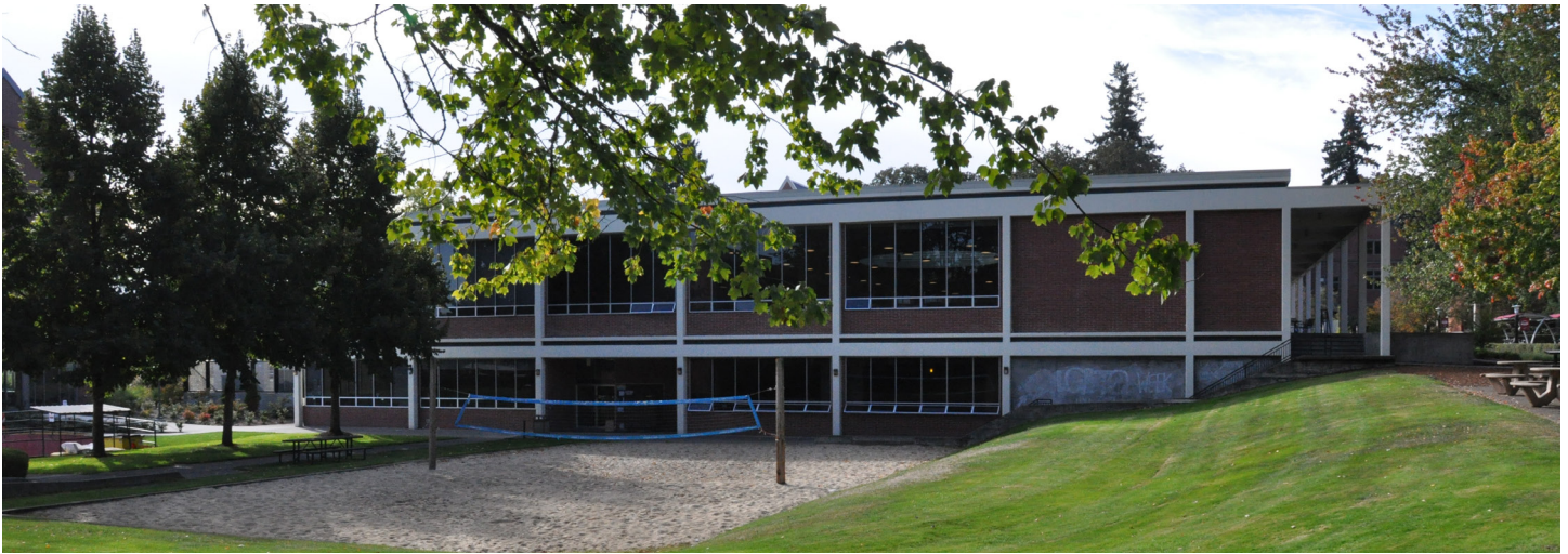
Figure II-3: The largest change proposed to the campus is demolition of Clark Hall and the conversion of the area north of the University Center to become a new north entry plaza to the campus. This will allow the University Center (above) to better serve as a welcome center and hub for students.
