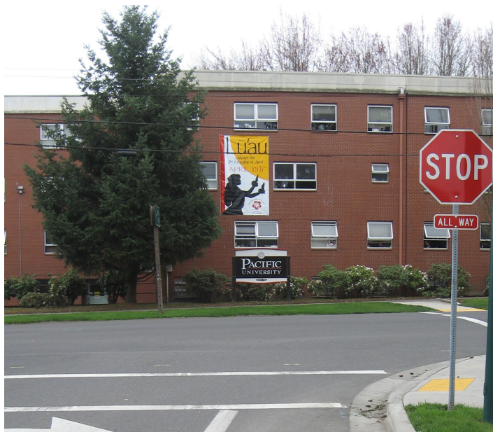
Figure IV-11: Demolition of Clark Hall to allow creation of a North Entry Plaza is a top priority under this planning cycle. The intent is to create a welcoming entry from the intersection of Sunset Drive and University Avenue.
