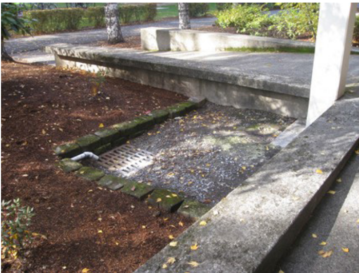
Figure VII-15: Existing catch basin at the University Center offers a stormwater planting opportunity (Mayer/Reed)
