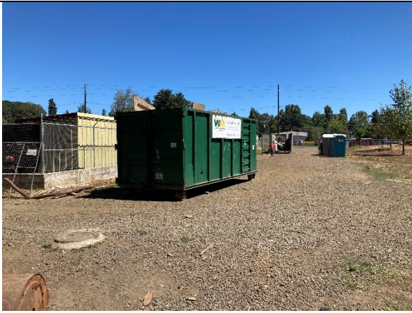
Description: Dumpsters placed on 1 st day of cleanup.
