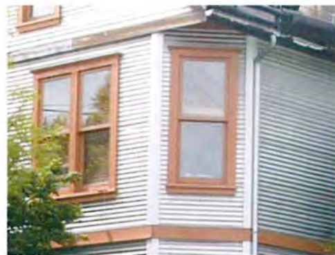
Well-Crafted Matching Wood Window Replacement Inappropriate Siding and Trim Replacement
