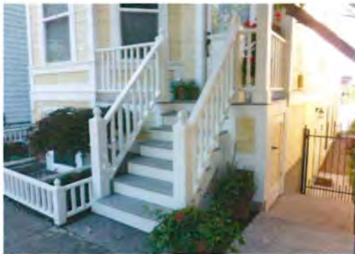
Example of a Single-Story Cottage Raised 3 Feet to Allow Lower Level Improvements; the Historic Relationship to the Ground is Retained
