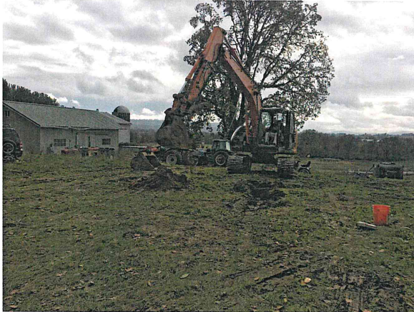
Test Pit TP-7
