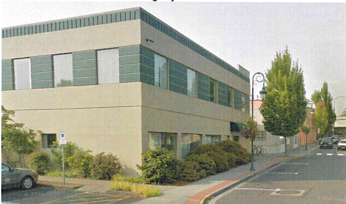
Existing City Hall Facade
