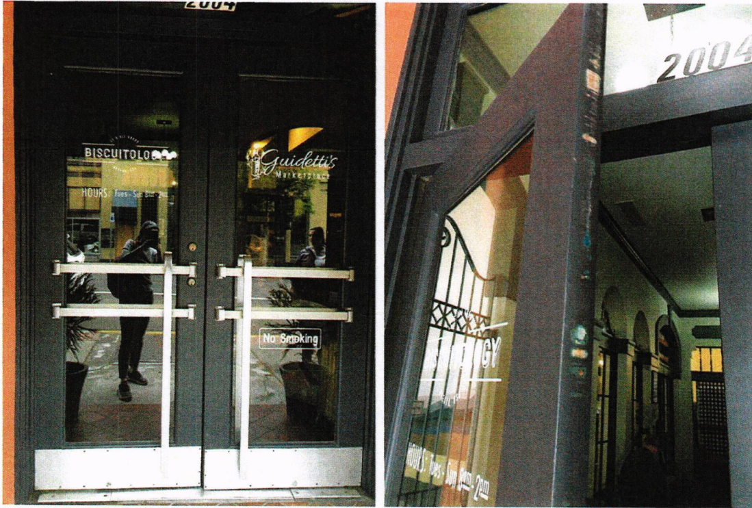
Figure 3. — Before Picture of Pacific Ave Main Entrance Doors. Worn hinges causes doors to not close properly. Left image shows that the door frames scrape against each other.
